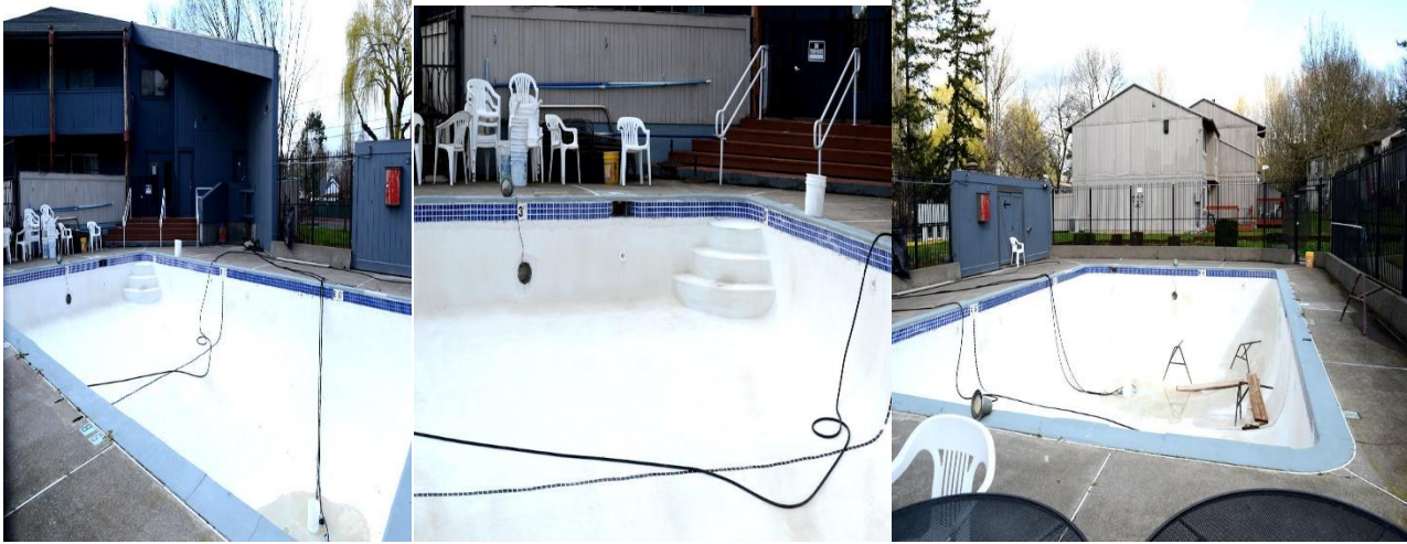
Pictures of the restoration process.
